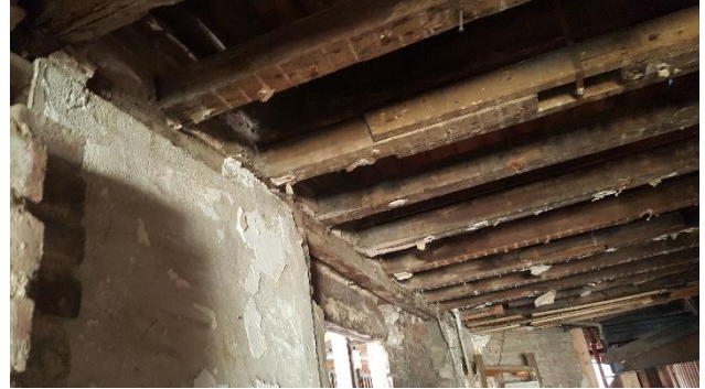
JOISTS OVER OPENING WITHOUT LINTEL. DEFLECTION OF SILL BEAM
