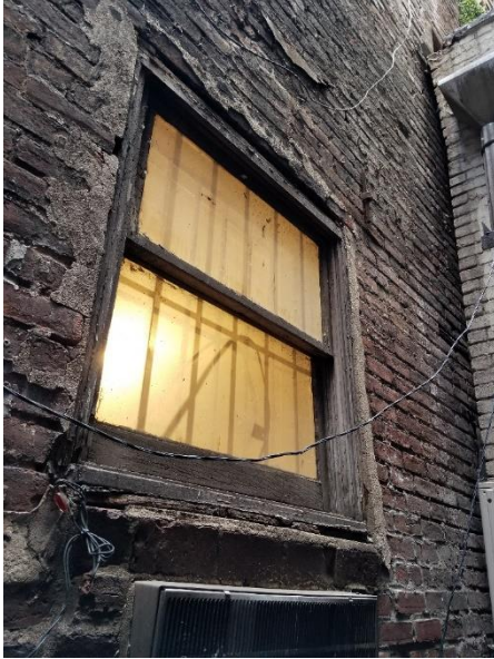
SILL AND LINTEL IN VERY POOR CONDITIONS AT BOTTOM WINDOW SIDE FAÇADE
