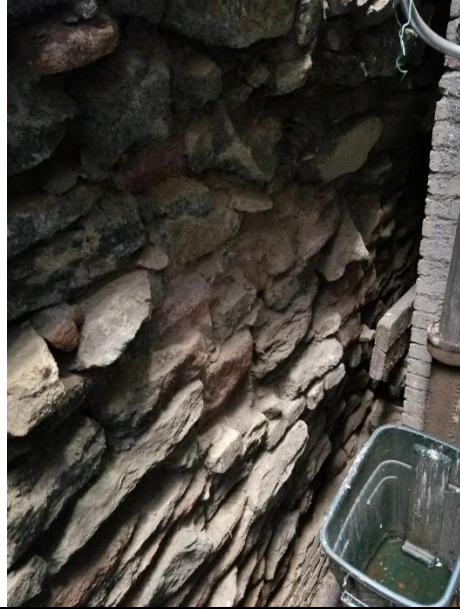
275 BLEECKER FOUNDATION WALL OUTSIDE FACE IN GOOD CONDITIONS
