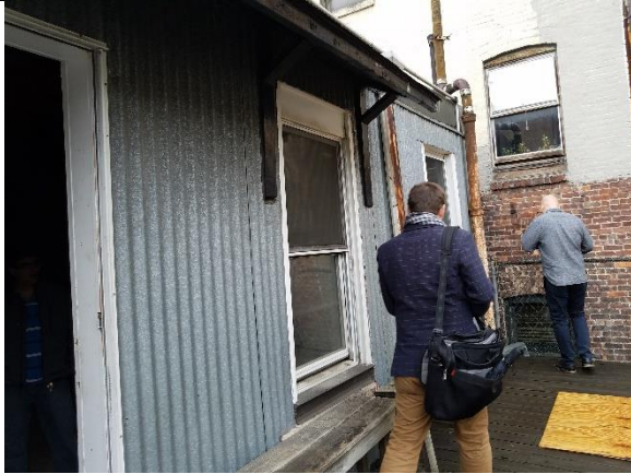
REAR FAÇADE FOURTH FLOOR CORRUGATED STEEL
