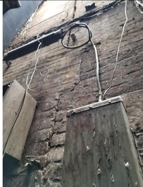
VERTICAL MEDIUM CRACK AT 275 BLEECKER SIDE FAÇADE
