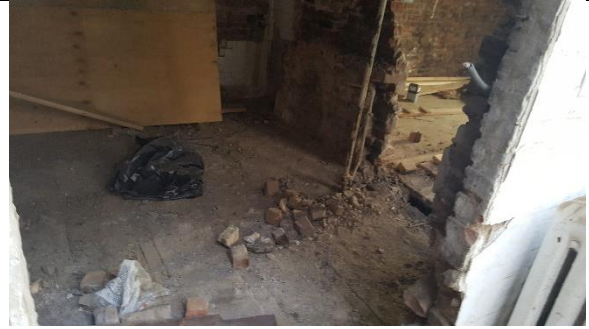
JOISTS OVER OPENING WITHOUT LINTEL. DEFLECTION OF SILL BEAM
